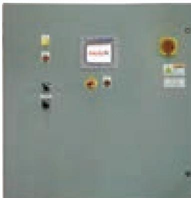
**AutoJet Spray Control Panel** provides easy control of nozzles and controls the liquid flow for both the binder solution and the fragrance.
